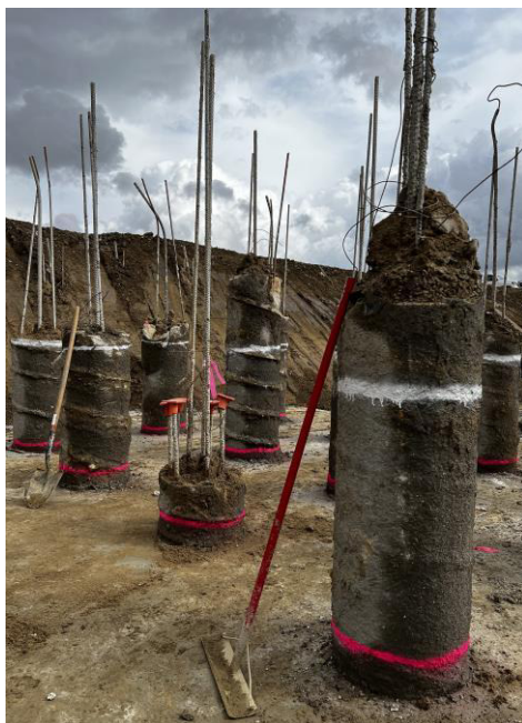
Fig. 14. Excavated Piles to be Chipped to Final Cut-off Levels
